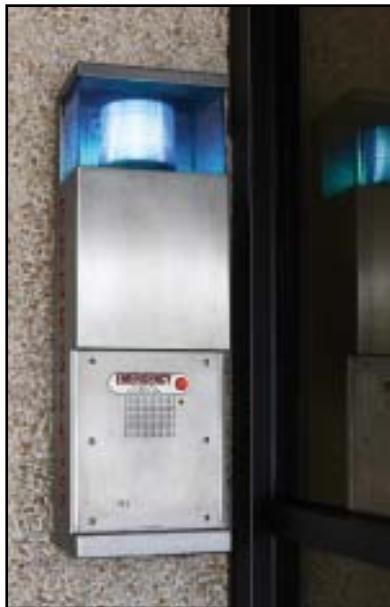
BCD Voltage Systems was commissioned to replace the existing telecommunications wiring along with emergency phones. City of Phoenix selected Talk-A-Phone's line of phone line powered emergency phones for this installation.
